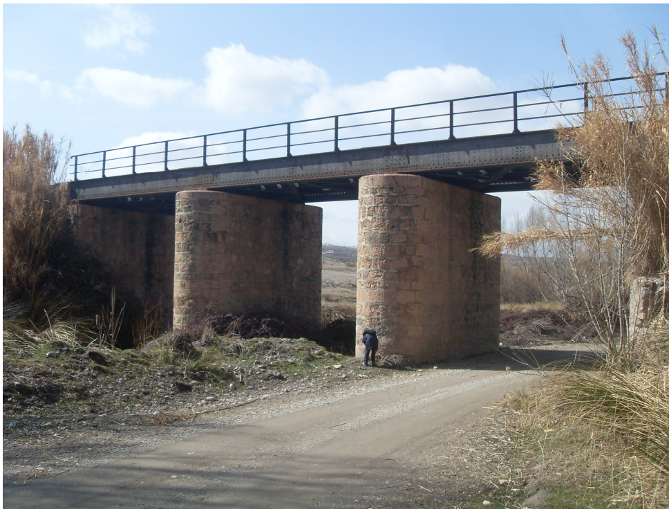
Figure 11: The definitive Gor bridge, 1909. Three 5,60 m continuous spans. Photograph by the authors.
