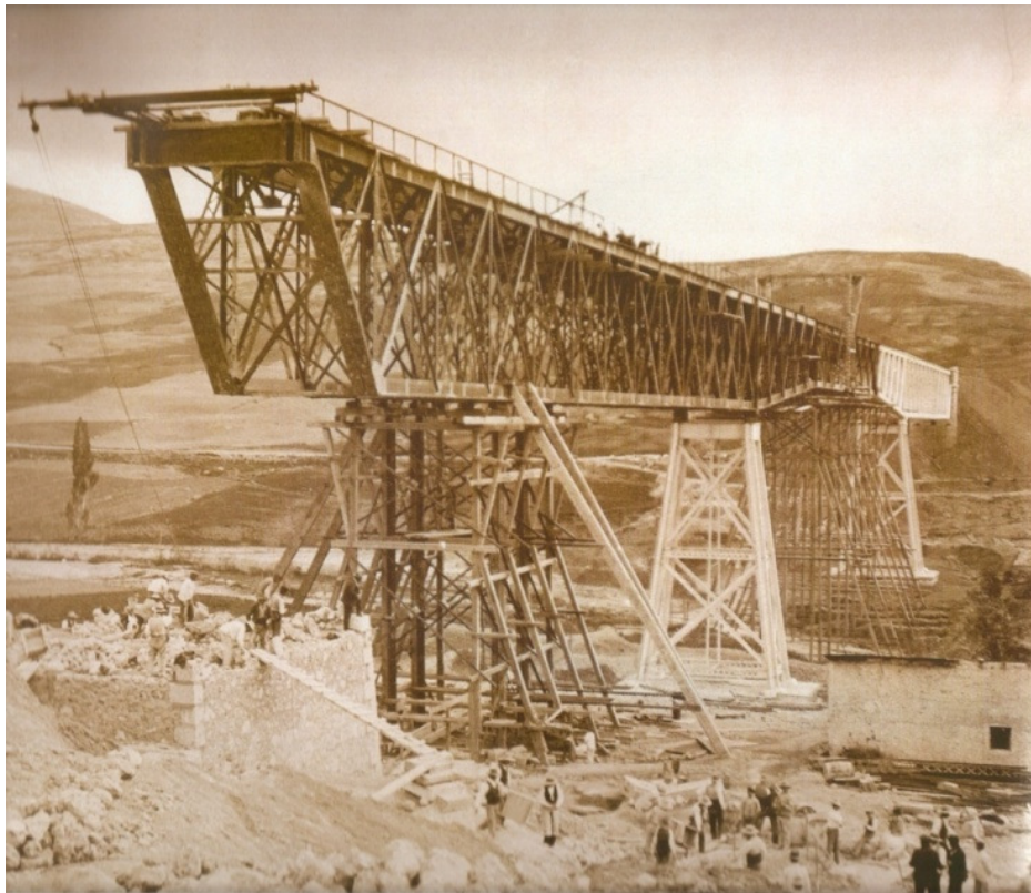
Figure 9. Works to build the new abutment, Winter 1906. Workers are demolishing the old abutment, while the viaduct is provisionally resting on trestles. Photo by Gustave Gillman, 1906. Courtesy of heirs of Gustavo Gillman.
