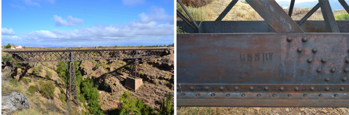
Figure 5: Baúl viaduct as finally built in 1904. Note the 'GSSR' marks on the bottom chord (detail). Photographs by the authors.
